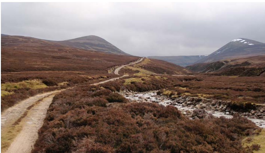
Fig. 3 First part of pipeline to be buried alongside existing track
