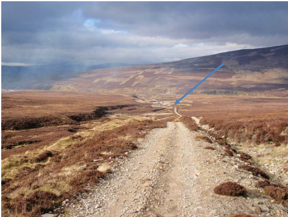
Fig. 8 - Route of pipeline looking back to Powerhouse and laydown area.
