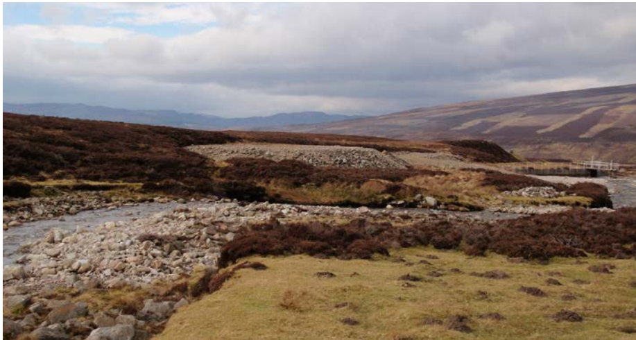
Fig. 2 – Turbine House location (existing intake in background right)
